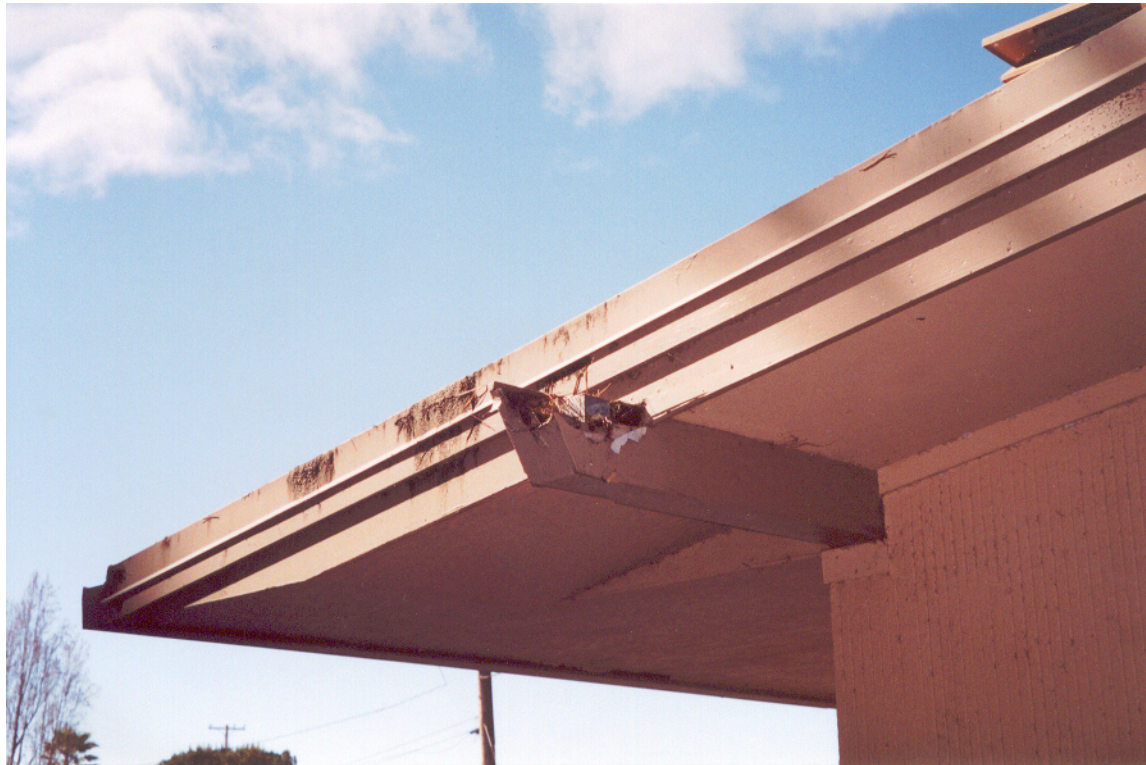
Figure 15: Deterioration of Roof Beam at Kindergarten Building
