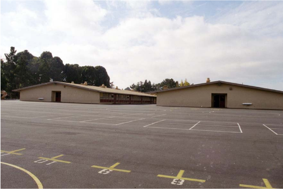
Figure 7: Northeast End of Classroom Buildings
