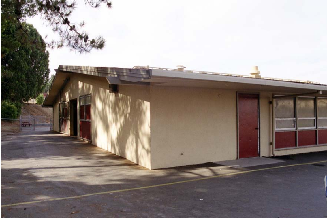
Figure 10: Southeast Face of Kindergarten / Library Building
