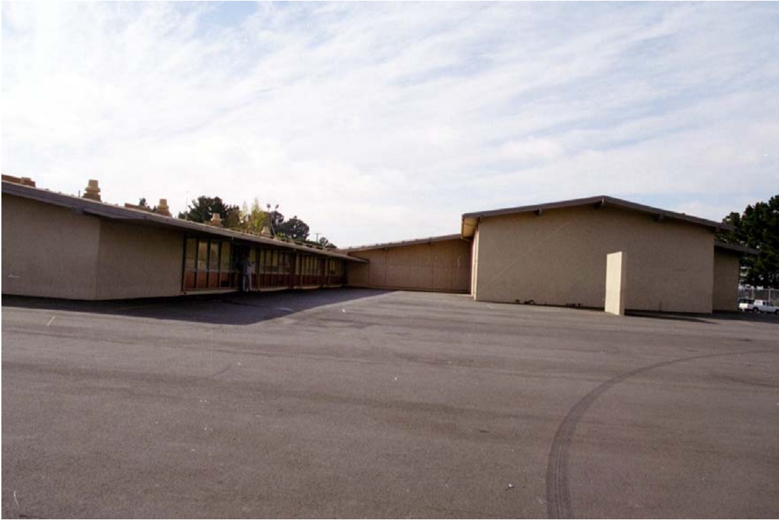
Figure 6: Rear of Multi-Purpose Building and Northwest Classroom Building
