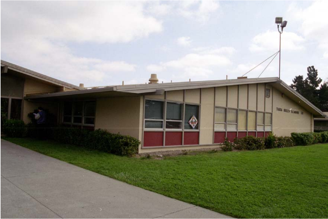
Figure 3: West Corner of Administration Area
