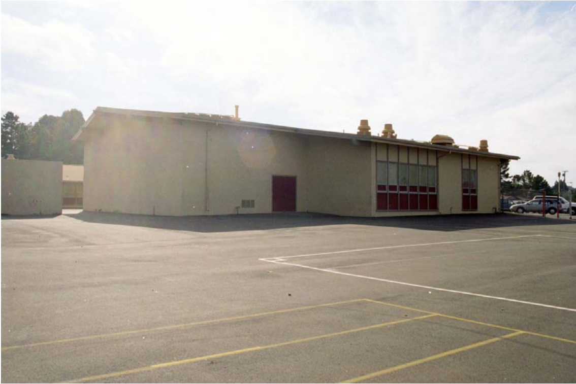
Figure 5: North Corner of Multi-Purpose Building
