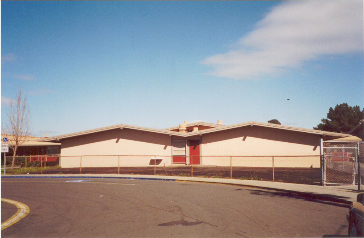
Figure 12: Southwest End of Southeast Classroom Building
